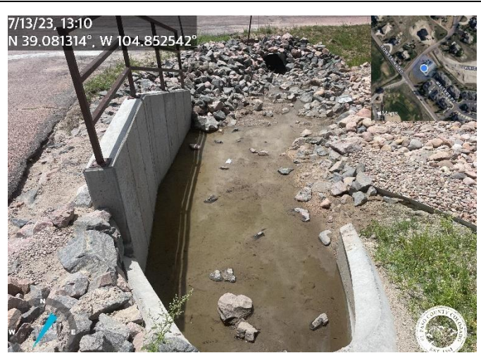
Photo 2: Install riprap apron at Leggins Way outfall of pond P4.
