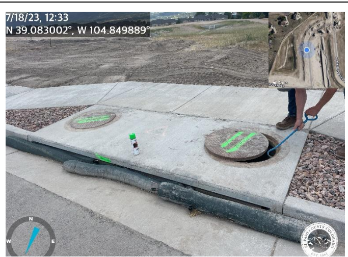
Photo 4: Remove forms and clean out above inlet painted with green strips.
