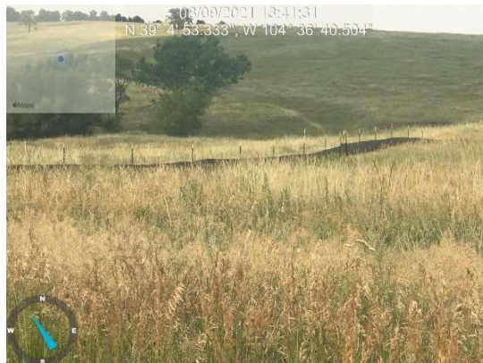
Silt fence implemented per plans around future pond.
