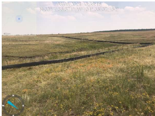
Initial control measures have been implemented per GEC plans.
