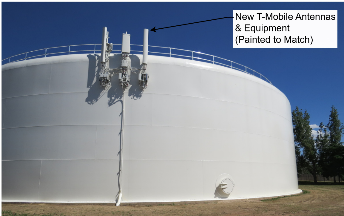
New View with New T-Mobile Antennas
