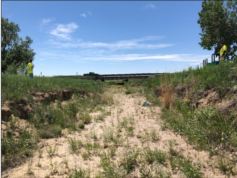
Figure 2-13. Priority Area 6 on East Fork Reach E2
