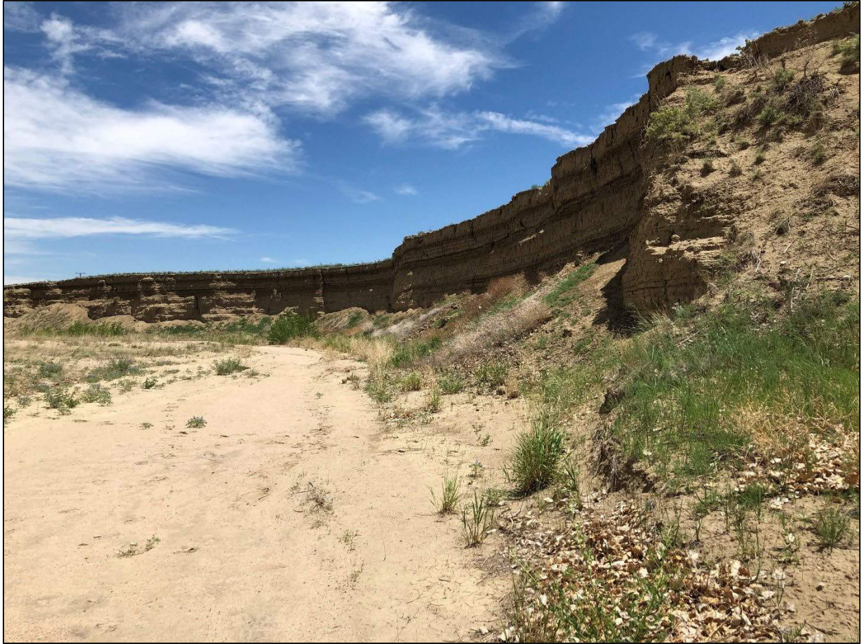
Figure 2-14. Priority Area 7 on Corral Tributary Reach C1
