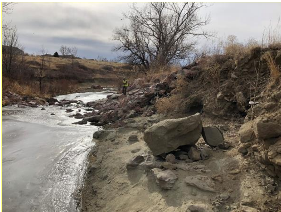
Figure 4-9. Example of degradation in Sand Creek near Barnes Road Bridge in Colorado Springs.
