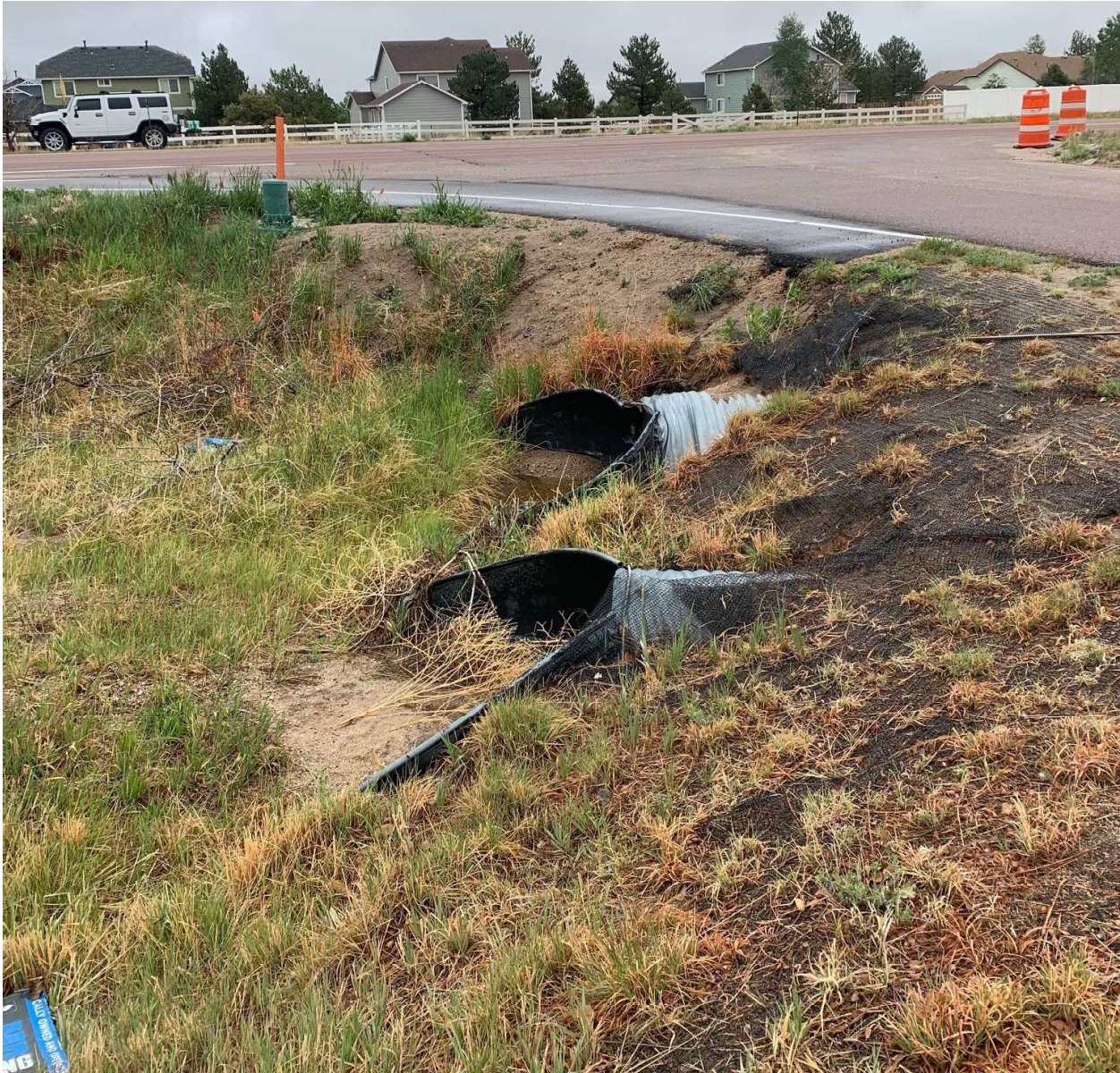
Existing 2-36" CMP under Owl Place (Upstream Inlets)
