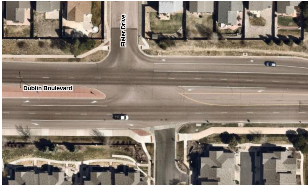
Dublin Boulevard & Fieler Drive
