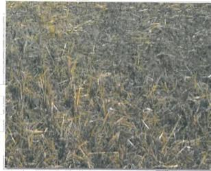
Mulch can be applied either using standard mechanical dry application methods or using hydromulching equipment that hydraulically applies a slurry of water, wood fiber mulch, and often a tackifier.
