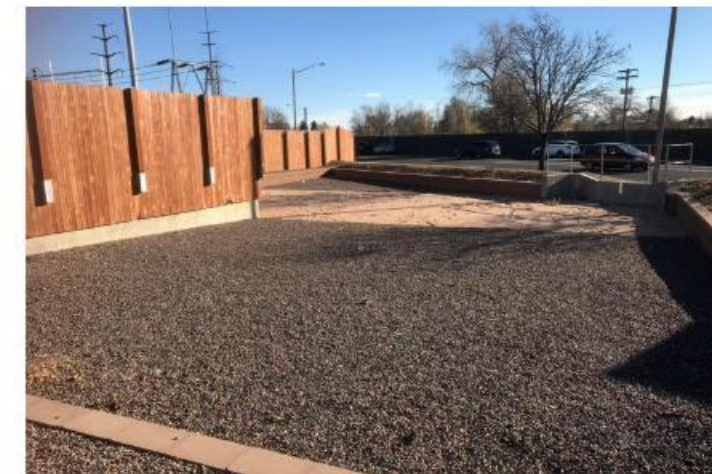
Photograph SF-3. Sand filter with incorporation of minor event flood attenuation provides water quality and detention for a substation.
