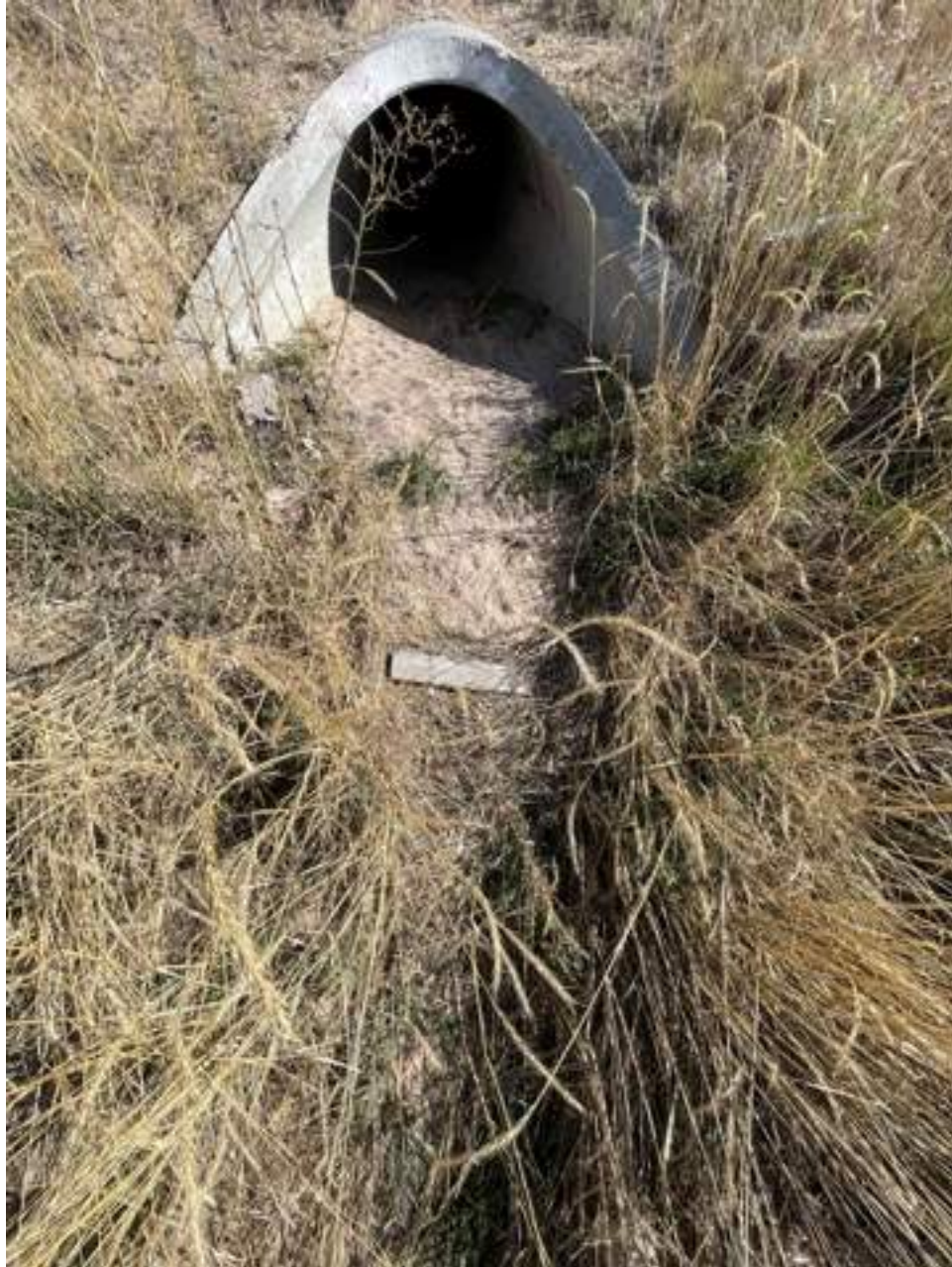
Figure 4: Outlets of pipes into the pond have built up with sediment over time and there is no energy dissipation installed. Type VL rip-rap is to be installed.
