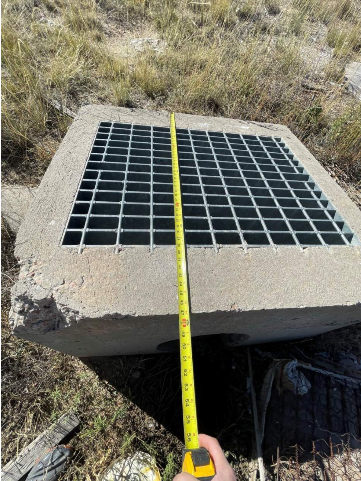
Figure 3: Measurements were taken to ensure that the outlet structure was constructed according to the Construction Drawings. A trash rack was installed per the detail.
