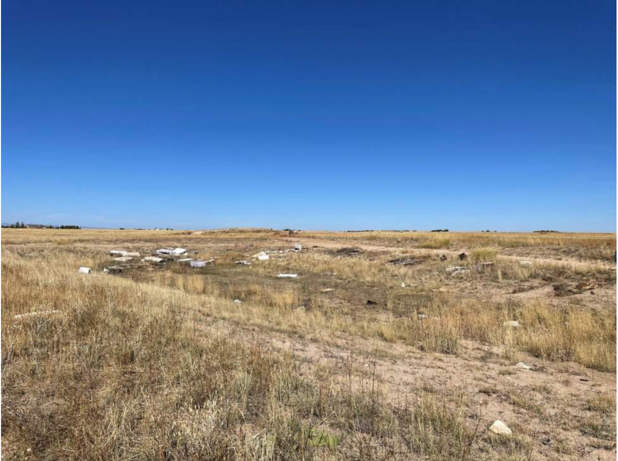
Figure 1: Existing Pond appears to have been constructed as designed in terms of topography. There is much debris to be disposed of as a part of this project.
