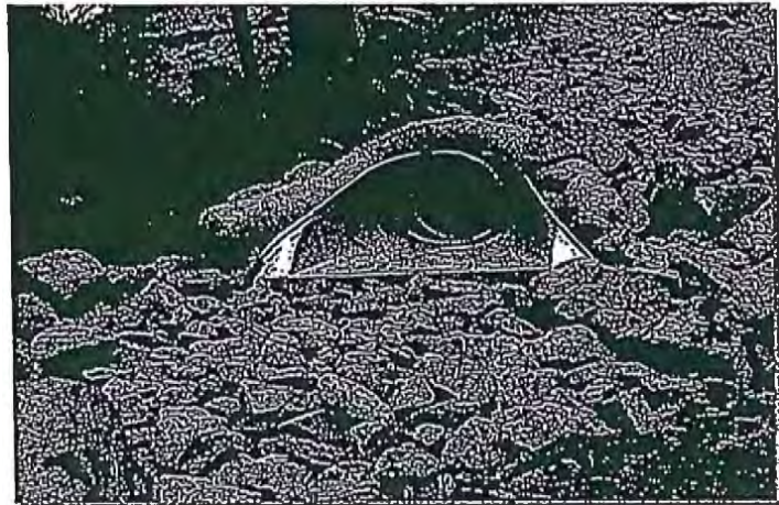
Photograph TOP-1. Riprap outlet protection.
