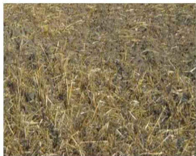
Photograph MU-1. An area that was recently seeded, mulched, and crimped.
