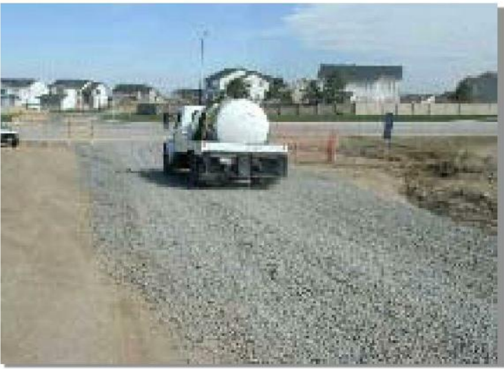
Photograph DC-1. Water truck used for dust suppression. Photo courtesy of Douglas County.
