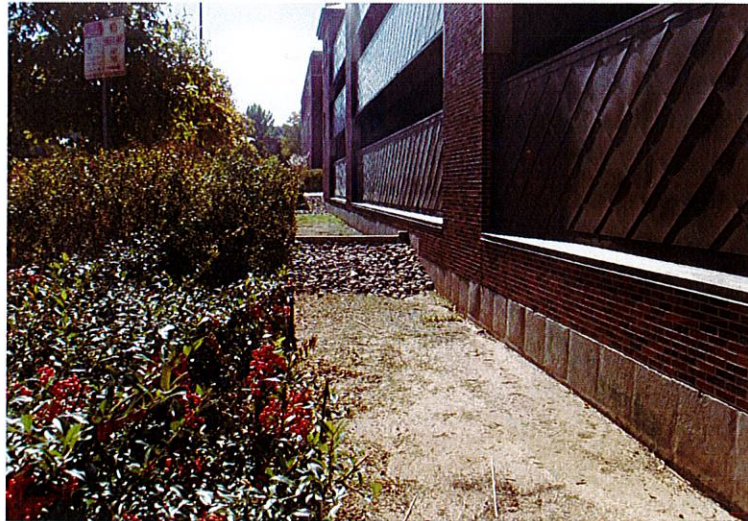
Photograph SF-1. This sand filter, constructed on two sides of a parking garage, is accessible for maintenance, yet screened from public view by a landscape buffer.
