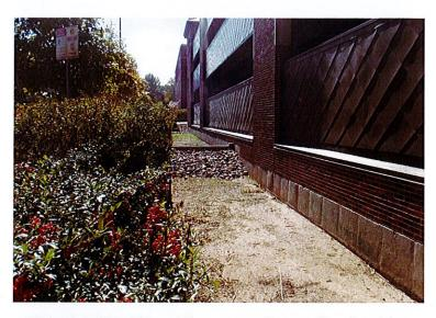
**Photograph SF-1.** This sand filter, constructed on two sides of a parking garage, is accessible for maintenance, yet screened from public view by a landscape buffer.
