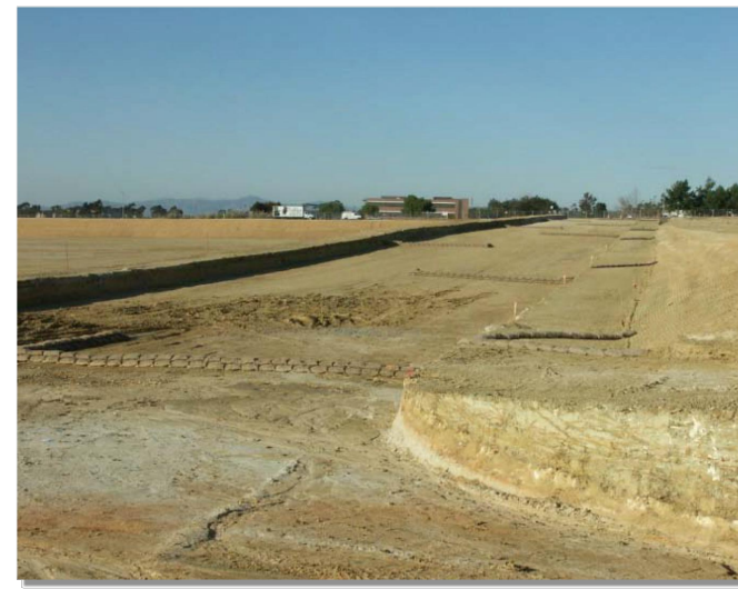
Photograph RCS-1. Rough cut street controls.
