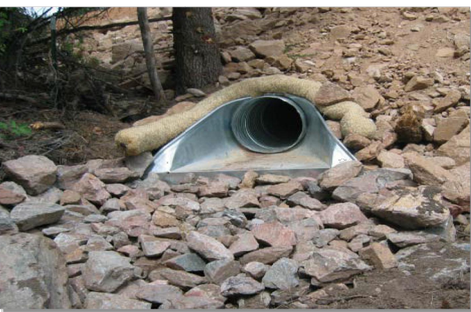
Photograph TOP-1. Riprap outlet protection.
