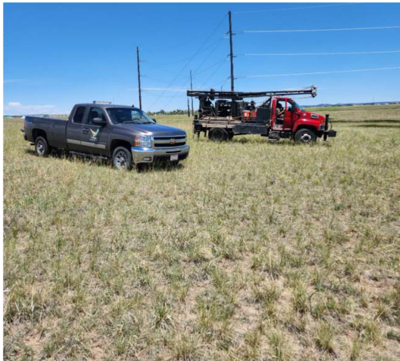
SITE CONDITIONS AT BORING B-11 - LOOKING NORTH
