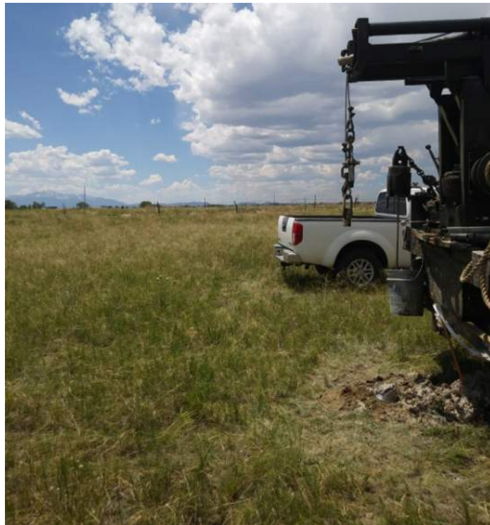
SITE CONDITIONS AT BORING B-2 - LOOKING WEST
