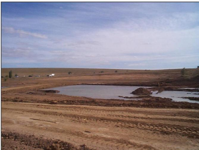
This low area will provide for some removal of sediment; however, it lacks a designed outlet structure.
