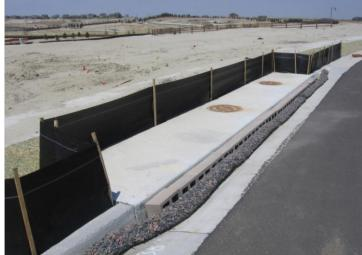
Photograph IP-1. Inlet protection for a curb opening inlet.
