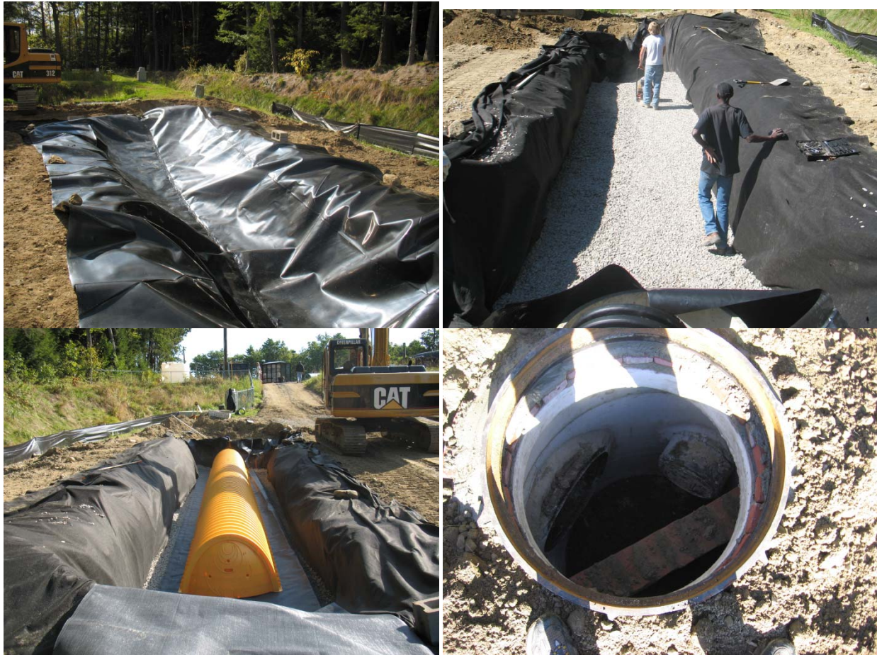
Figure 2: Installation of Isolator Row September 2006; (a, top left) HDPE liner installation to monitor full treated effluent; (b, top right) Crushed stone subbase 12” thick installation; (c, bottom left) Installation of Isolator Row chambers on top of double layer of woven geotextile fabric (bottom) non-woven geotextile fabric (sides) and stone subbase; (d, bottom right) Installation of hydraulic inlet structure, chamber entrance (left), influent source (top right), and high flow bypass weir bottom right.
