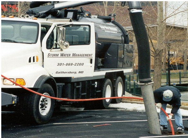
Figure 5: Vacuum truck and high pressure hose
