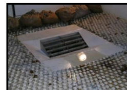
CDOT Type D Inlet Parallel (30° Incline & Depressed)
