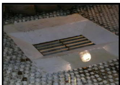
CDOT Type D Inlet Parallel (Flat & Depressed)
