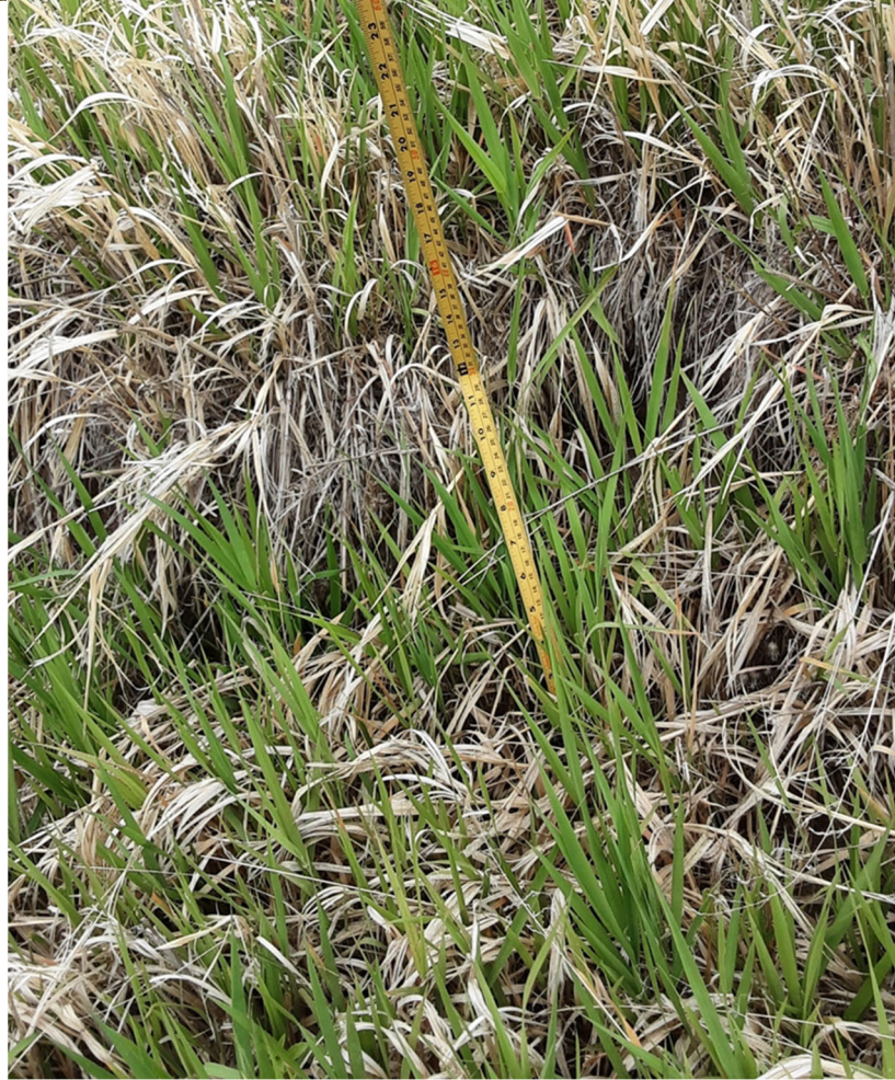
Figure 10: Erosion Found At Drainage Path 5 to 10 feet from East Property Line (Approximately 1-1.5 foot drop)
