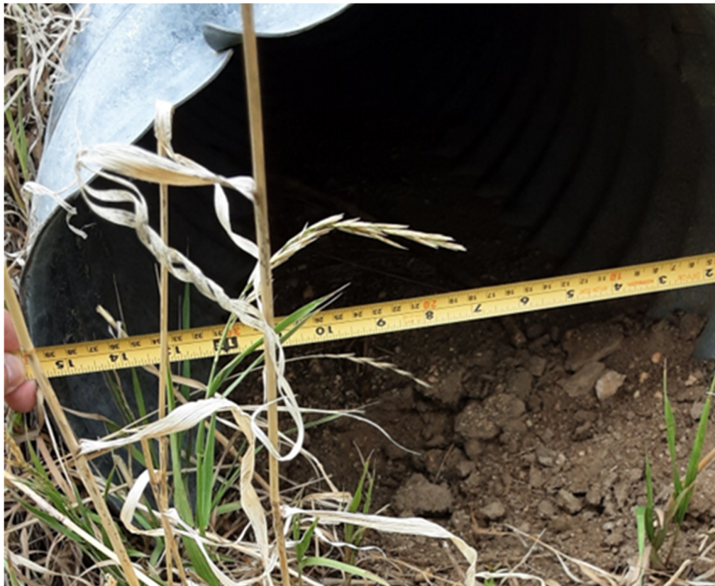
Figure 5: Measurement of Existing 15" Diameter Pipe
