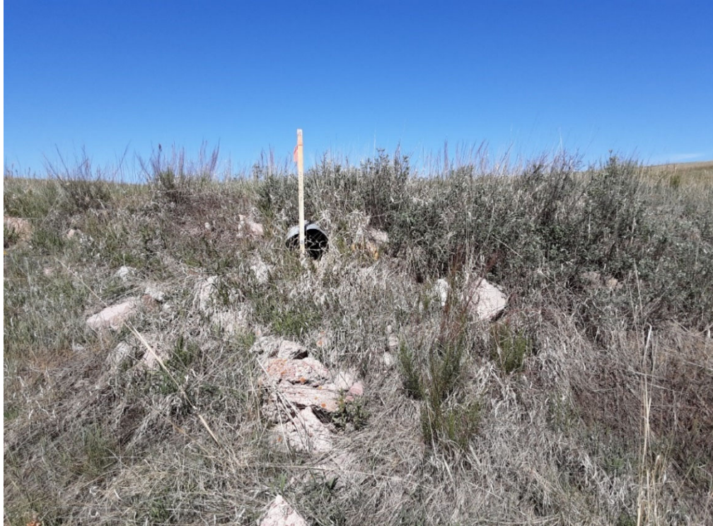
Figure 4: Existing 15" Diameter Spillway Pipe
