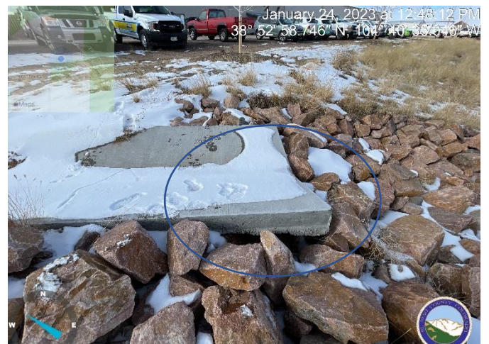
Photo 4: Concrete channel at southwest corner of pond is undercut. Voids need to be filled with non-erosive material as to not compromise structure.
