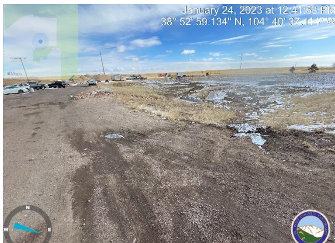
Photo 3: Storage lot/Gravel driveway. Top left corner adjacent to concrete lined forebay (North). Berm up top of slope. Bypassing causing erosion blowout.
