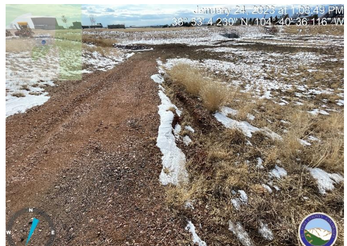
Photo 12: Maintenance access rd. Repair erosion rill atop of rd. Maintenance access rd. need to be redefined per detail. Reference sheet ST03 of GEC plan.
