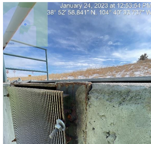
Photo 8: Trash screen bolts and nuts need to be replaced. Rusty and falling off structure.
