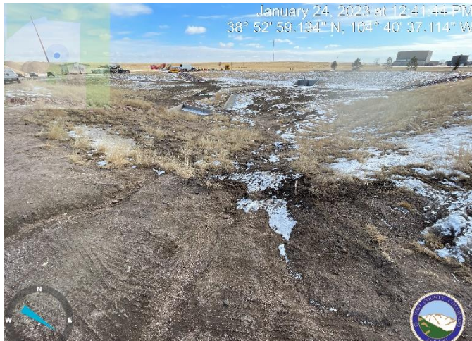
Photo 1: Storage lot/gravel driveway. Berm up top of slope of northwestern corner of pond embankment adjacent to concrete riprap rundown. Runoff is bypassing
