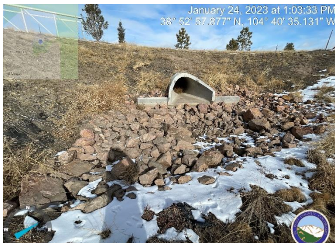
Photo 11: Low tailwater riprap basin. Plan detail calls for 24' L and measures 17' L in field. Reference sheet ST05A of GEC plan.
