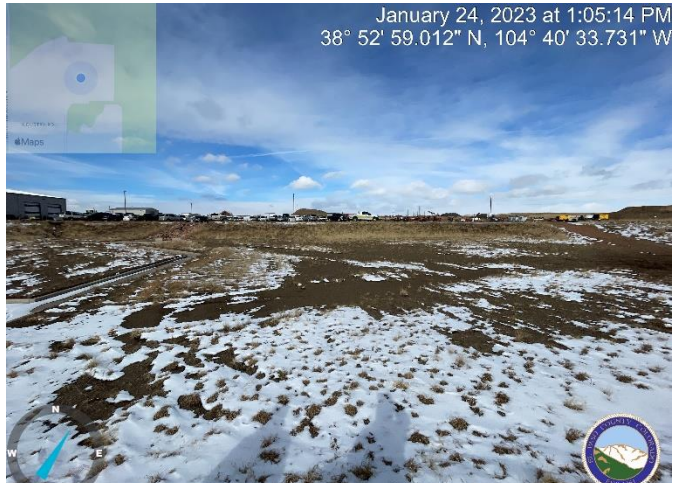
Photo 13: Sparse vegetation throughout bottom of pond structure. Sparse vegetation around pond outlet pipe. Seed did not take on steep slopes. TRM called for on
