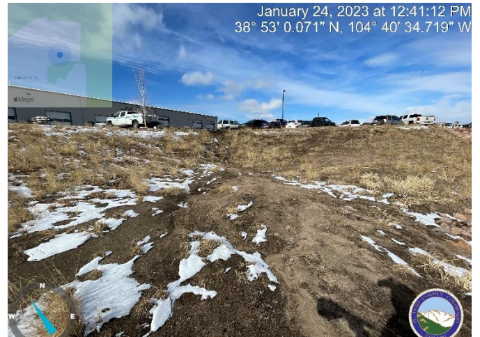
Photo 2: Subsequent sediment discharge from top of gravel parking lot into pond also needs to be cleaned out. Reference photo #1.
