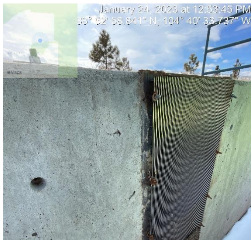
Photo 7: Gap between trash screen and concrete, needs to be flush.
