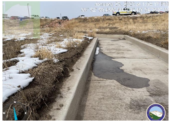
Photo 6: Pond bottom is above grade of low flow channel top of curb. Bring grade down to match top of curb, at 4% min slope per sheet ST05.
