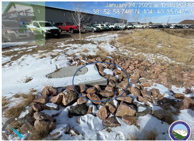
Photo 5: Concrete channel at southwest corner of pond is undercut. Voids need to be filled with non-erosive material as to not compromise structure.
