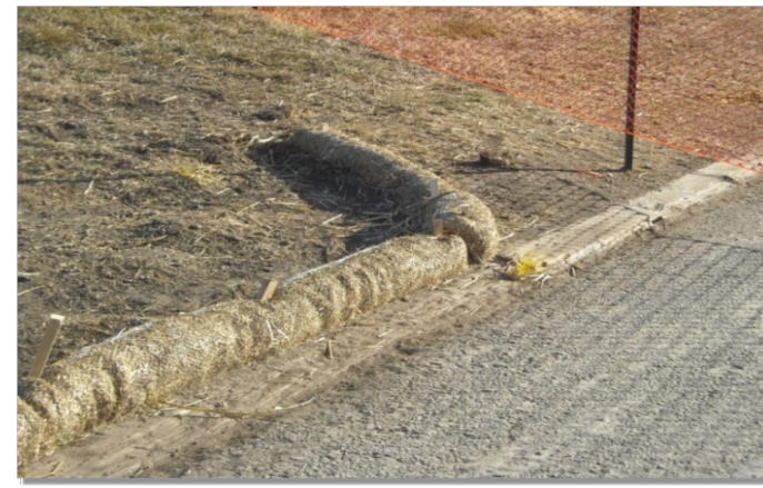
Photographs SCL-1 and SCL-2. Sediment control logs used as 1) a perimeter control around a soil stockpile; and, 2) as a "J-hook" perimeter control at the corner of a construction site.
