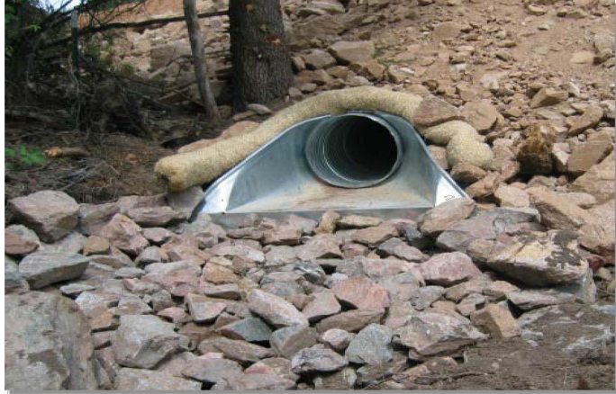
Photograph TOP-1. Riprap outlet protection.
