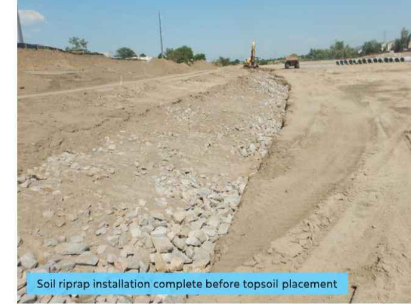
Soil riprap installation complete before topsoil placement
