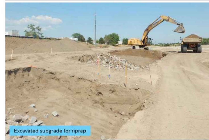
Excavated subgrade for riprap
