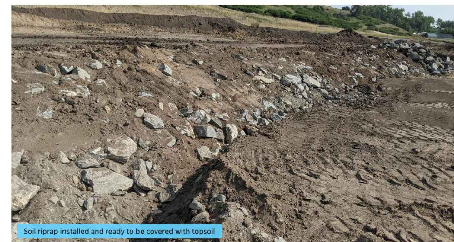
Soil riprap installed and ready to be covered with topsoil
