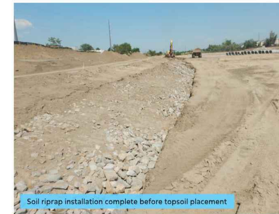
Soil riprap installation complete before topsoil placement
