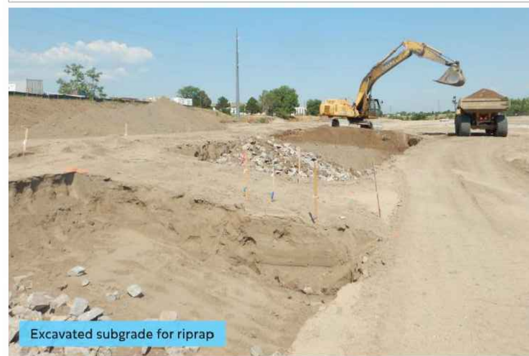
Excavated subgrade for riprap
