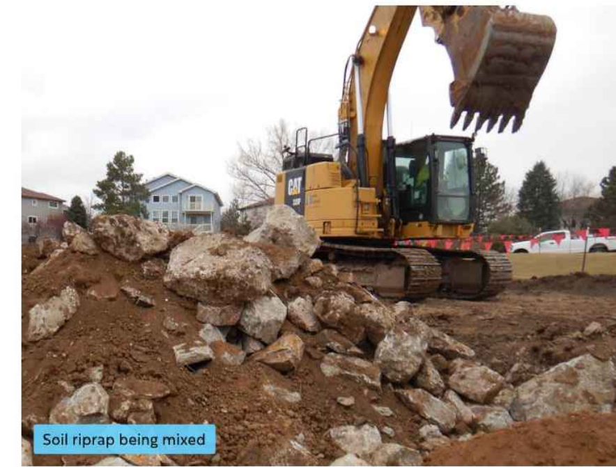
Soil riprap being mixed
