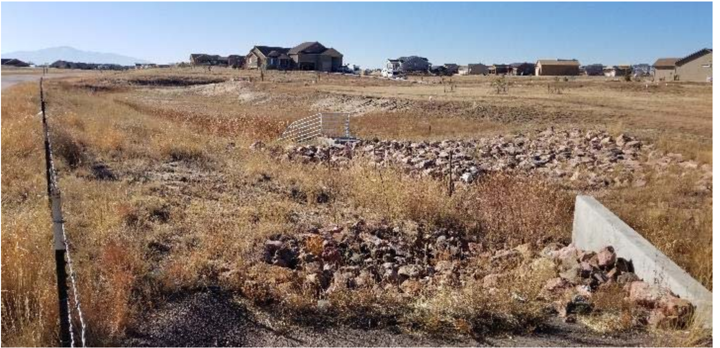
PP10 – SITE OVERVIEW FROM SOUTHWEST CORNER (LOOKING WEST)
