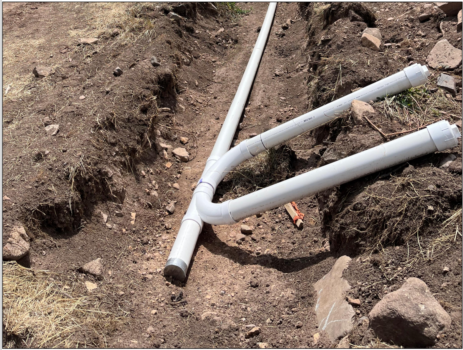
Typical Double Sweep Cleanout with Screw Cap
