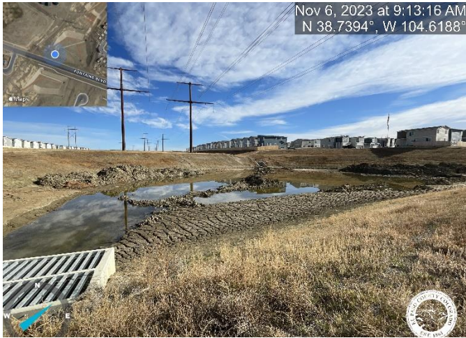
Photo 11: Pond C2.2: Repair damage to trickle channel curb approximately 30 feet from Forebay 'B'. Item will be checked once pond is cleaned.
