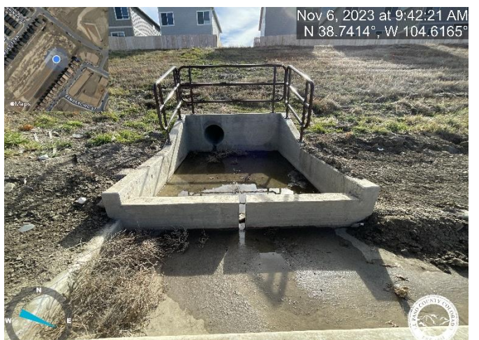
Photo 20: Pond C3: Remove debris and sediment from forebays, trickle channel and outlet structure micropool.
