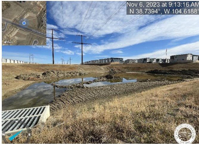
Photo 12: Pond C2.2: Grade pond bottom to match approved specs and Reinstall maintenance access road per plans. Plans call for 12" deep road base.
