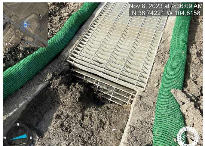
Photo 24: Pond C4: Remove debris and sediment from outlet structure micropool.
