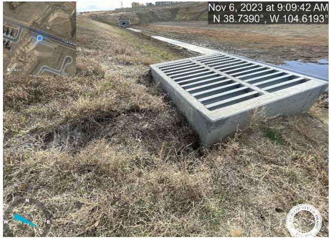
Photo 18: Pond C2.3: Backfill and stabilize erosion behind outlet structure.
