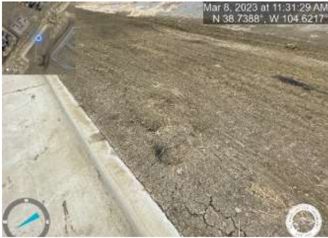
Photo 5: Pond C1: Remove old/damaged straw wattles from pond bottom.
