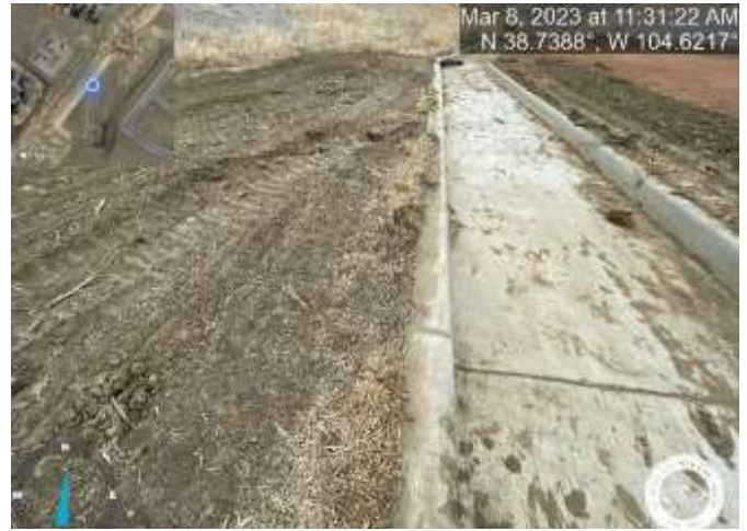
Photo 6: Pond C1: Remove old/damaged straw wattles from pond bottom.
