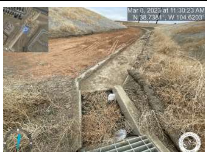
Photo 2: Pond C1: Remove excess sediment and old straw wattles from trickle channel.
