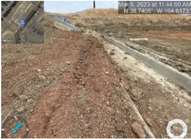
Photo 21: Pond C3: Remove road base from east perimeter of trickle channel near outlet structure.
