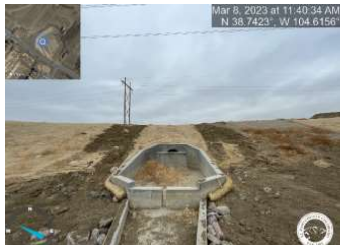
Photo 28: Pond C4: Reinstall erosion control blankets along pond slopes.
