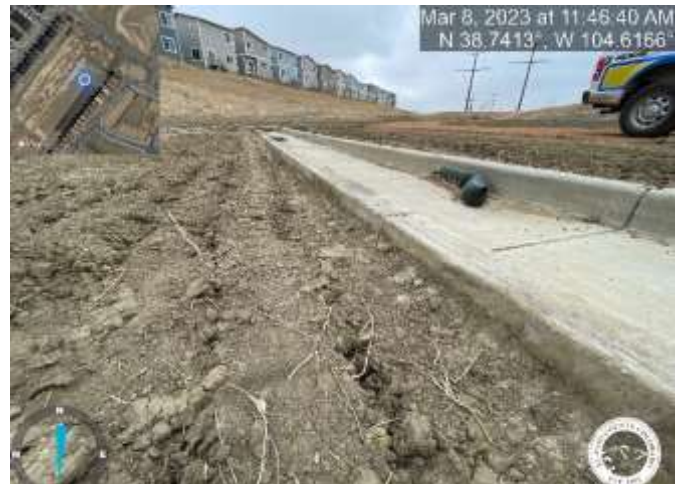
Photo 24: Pond C3: Raise pond bottom to top of trickle channel curb with a 3% slope towards trickle channel for positive drainage.
