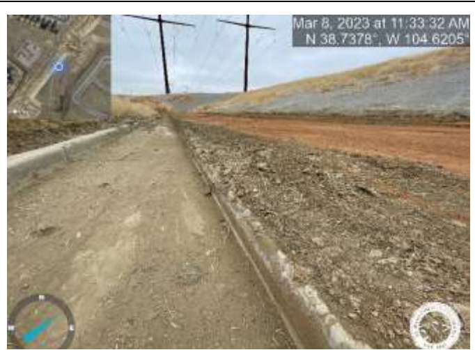
Photo 4: Pond C1: Remove sediment to match the top of trickle channel curb with a 3% slope towards trickle channel for positive drainage.
