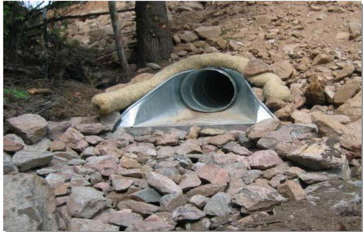
**Photograph TOP-1.** Riprap outlet protection.
