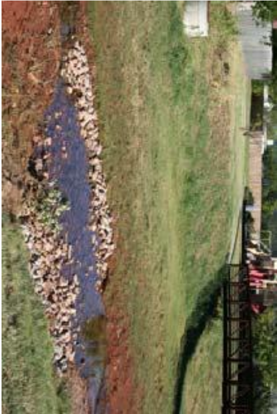
CONSTRUCTED RIFFLE DROP STRUCTURE
