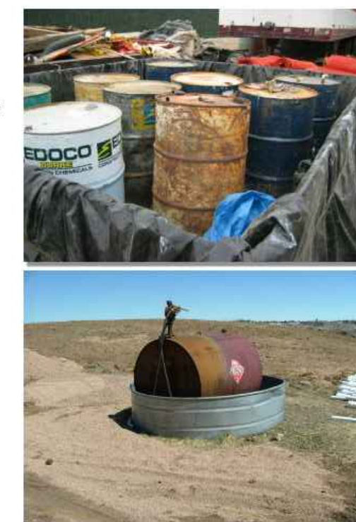
Photographs GH-1 and GH-2. Proper materials storage and secondary containment for fuel tanks are important good housekeeping practices. Photos courtesy of CDOT and City of Aurora.
