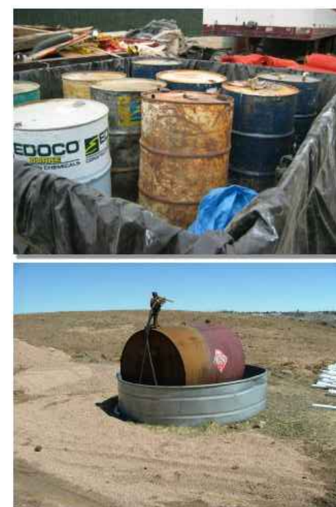
Photographs GH-1 and GH-2. Proper materials storage and secondary containment for fuel tanks are important good housekeeping practices. Photos courtesy of CDOT and City of Aurora.
