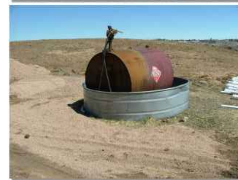
Photographs GH-1 and GH-2. Proper materials storage and secondary containment for fuel tanks are important good housekeeping practices. Photos courtesy of CDOT and City of Aurora.
