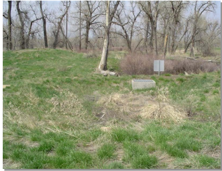
Photograph SF-1. The vegetation on the surface of the filter and the shallow design depth of this sand filter, help the BMP blend into its surroundings. Photo courtesy of Fred Bromberger.
