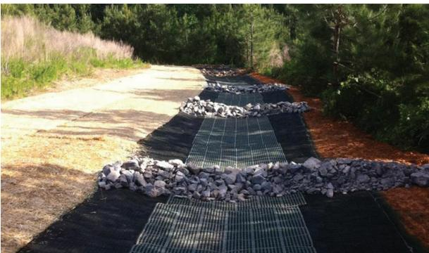
*To boost performance of the VMax turf reinforcement mats in critical applications, combine with our ShoreMax® flexible transition mat to create a system that can dramatically elevate the permissible shear stress and velocity protection beyond many hard armor solutions.*
