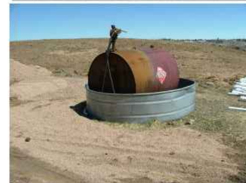
Photographs GH-1 and GH-2. Proper materials storage and secondary containment for fuel tanks are important good housekeeping practices.
