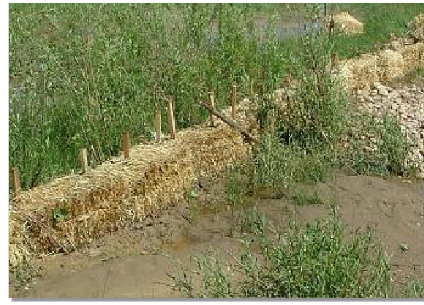
Photograph SBB-1. Straw bale barrier used for perimeter control. Photo courtesy of Tom Gore.
