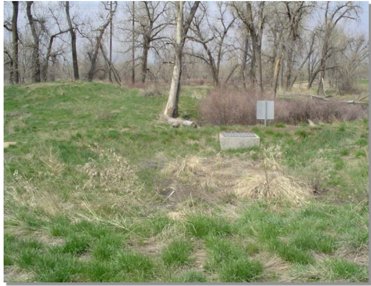
Photograph SF-1. The vegetation on the surface of the filter and the shallow design depth of this sand filter, help the BMP blend into its surroundings. Photo courtesy of Fred Bromberger.
