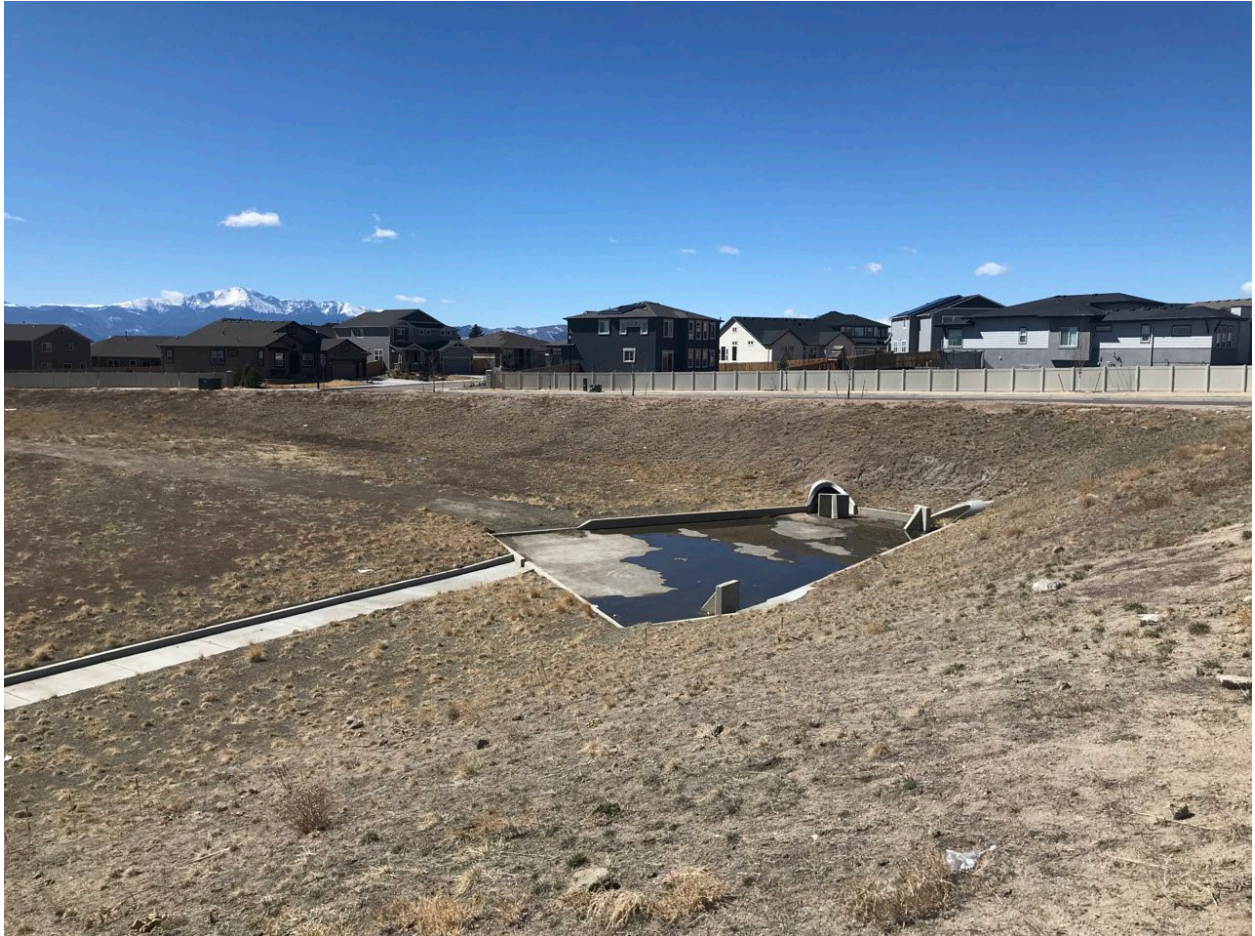
Photo Location 03. Looking southwest at stormwater facilities under residential development.
