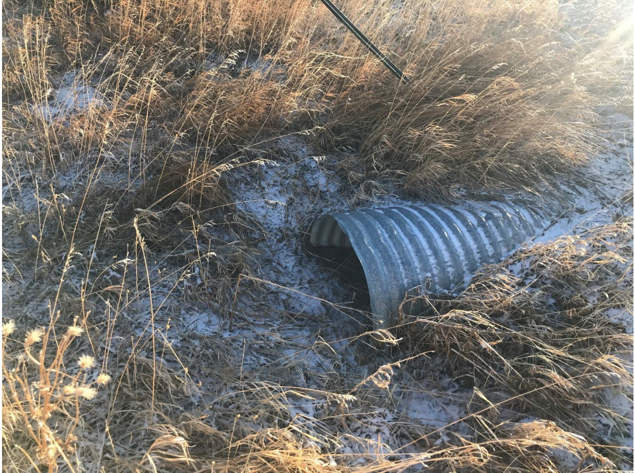
Photo Location 15. Culvert inlet near WT-A38 directed southeast offsite under Vollmer Road.
