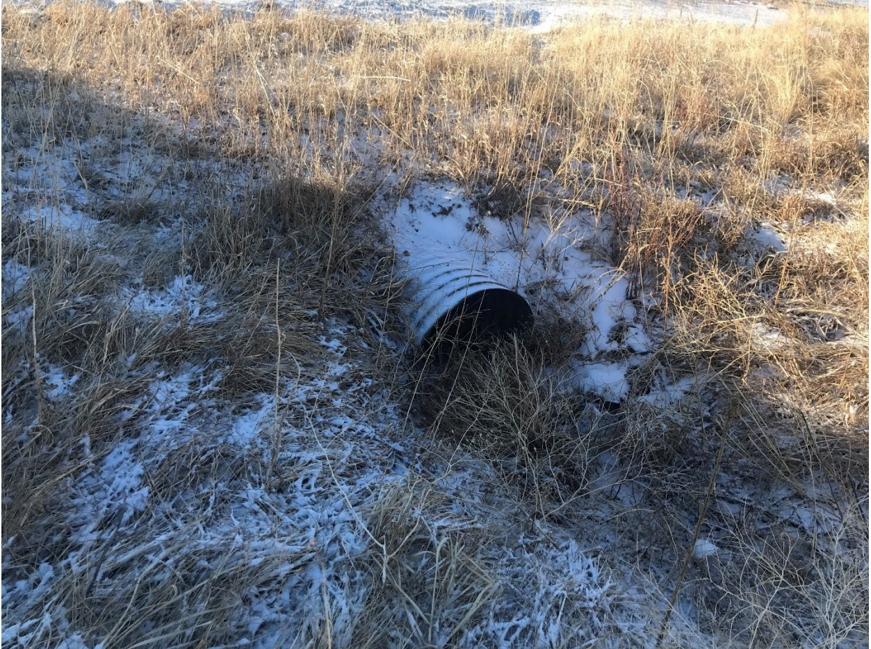
Photo Location 14. Culvert inlet near WT-A33 directed southeast offsite under Vollmer Road.
