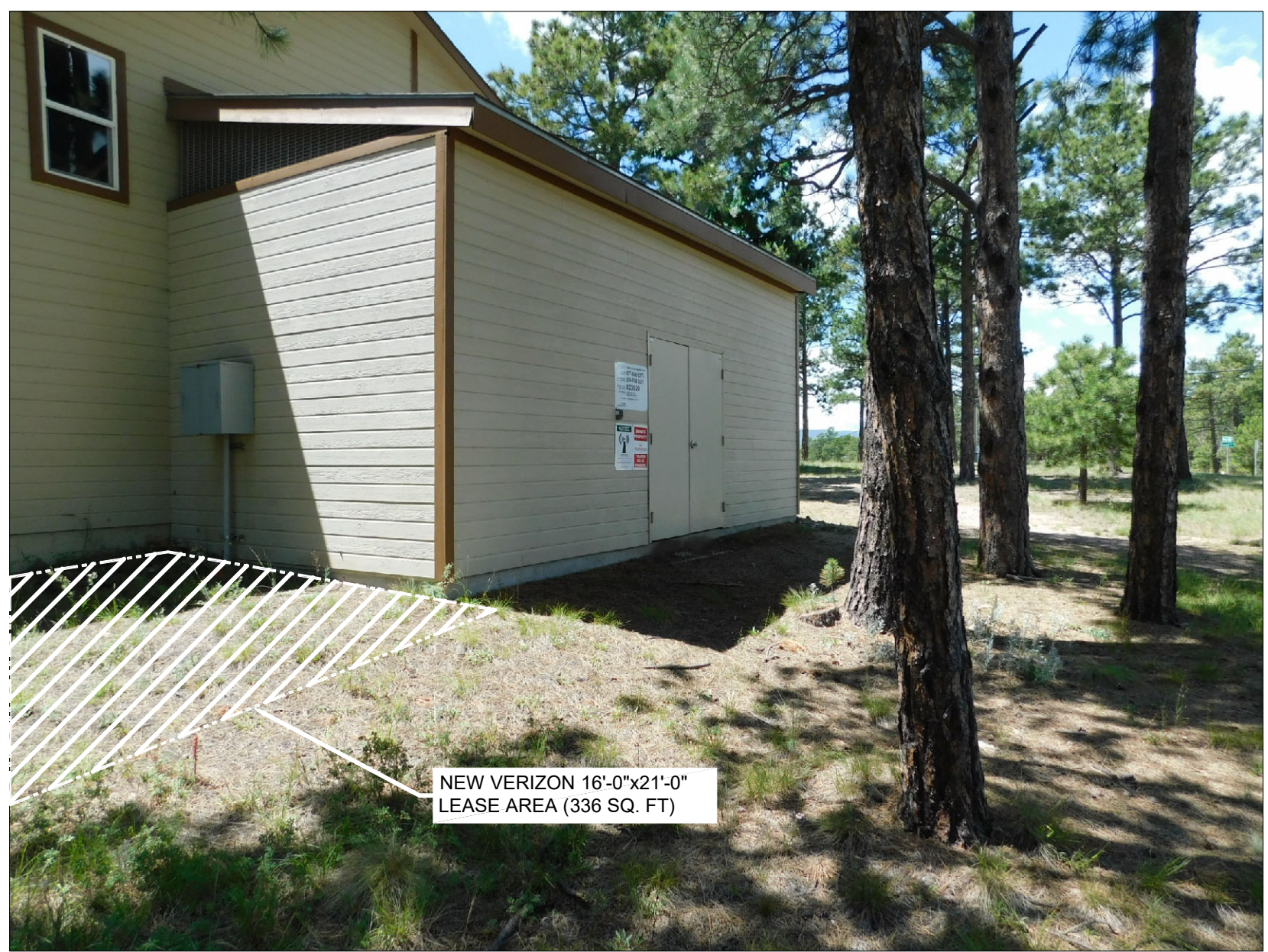
VIEW OF NEW LEASE AREA (LOOKING NORTHEAST)
