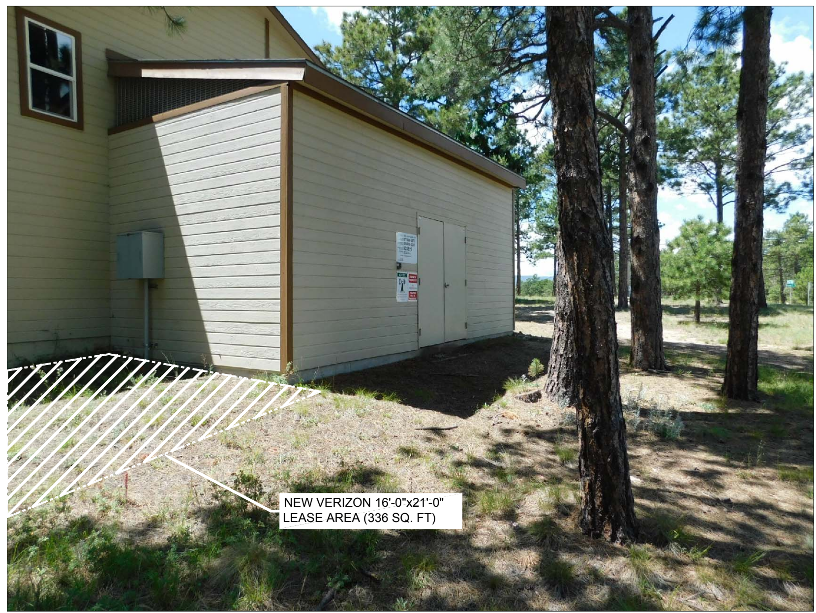
VIEW OF NEW LEASE AREA (LOOKING NORTHEAST)
